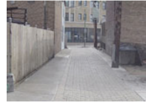
Alley with permeable pavement
