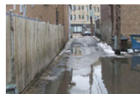
Alley prior to improvements
